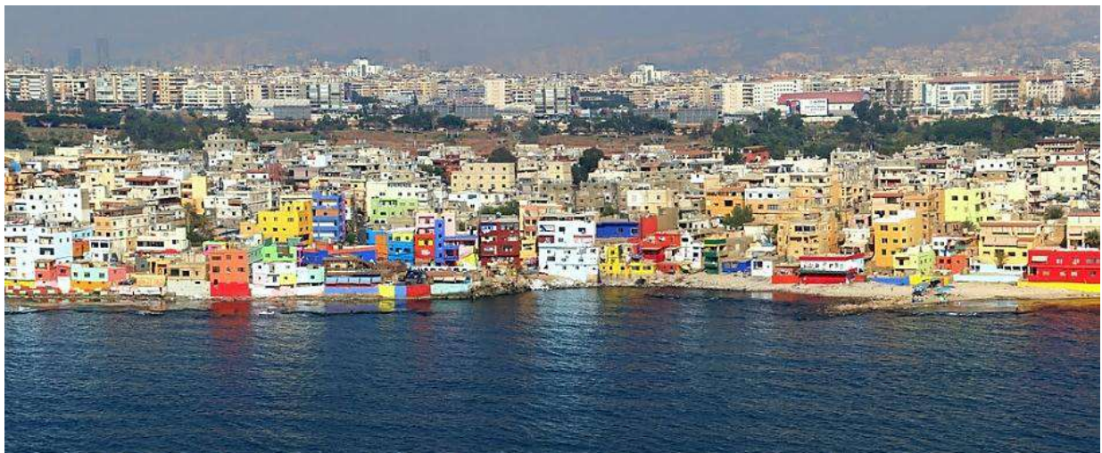
Fig. 10 The colorful façade of Ouzai Ouzville port. Photo: Getty Images.
