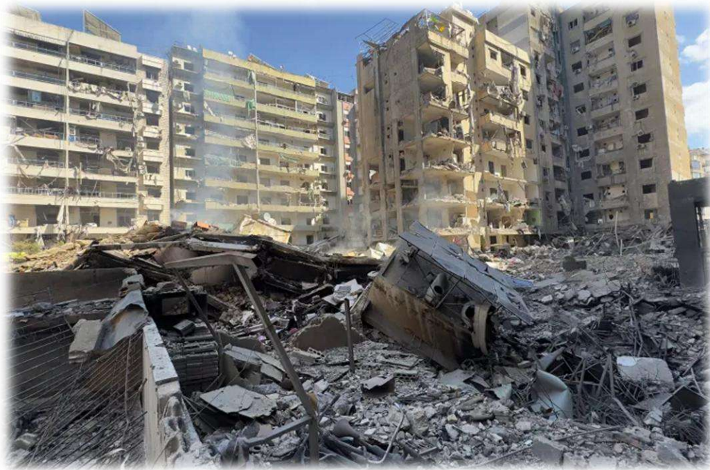
Fig. 4 Devastating destruction of various buildings in Dahiyeh. Photo: Aljazeera.
