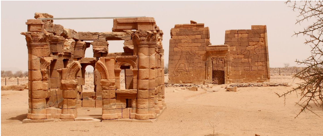
Condition of Naqa Monuments (February 2024)
